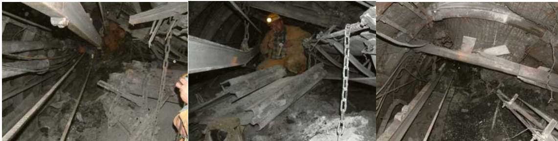
Figure 5 - Picture of rock burst effect in tunnel after tremor with seismic energy 9-107 J, ( M_L=3.3 ), which occurred on April 16th 2008. The gallery was damaged on segment of 85 meters and the floor was lifted up 1,5 m.
