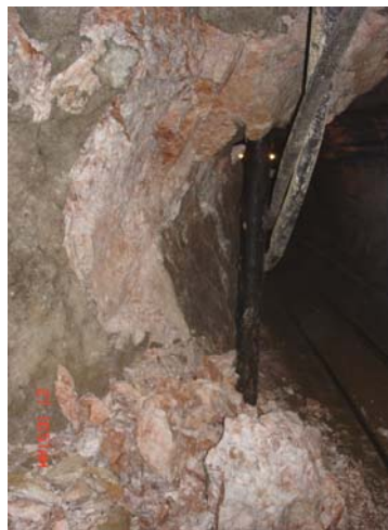
Figure 3 Schistose scaling on sidewalls in tunnel
