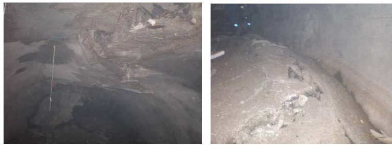
Figure 2 Rock deformation and fracturing situation after previous common bolting support
