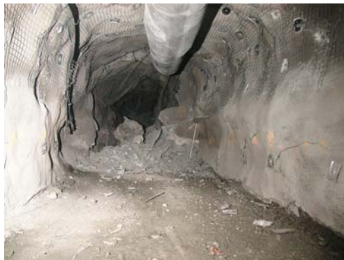
Figure 2 A 2.0 local magnitude seismic event during development of an ore drive
