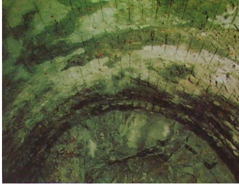
Figure 5 Full section excavation of circular tunnel
