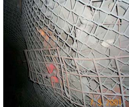
(b) Finely shattered rock contained by mesh [3]
