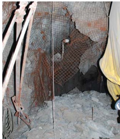
Figure 3 Roof collapse following a powerful seismic event in a deep mine.
