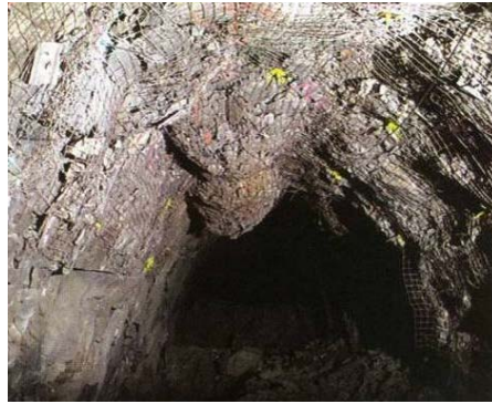
(a) Contained damage in the roof [2]
